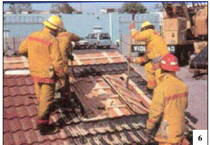
A "Lower" cut (shown here) opens a roof for ventilation without having to remove the roofing.
