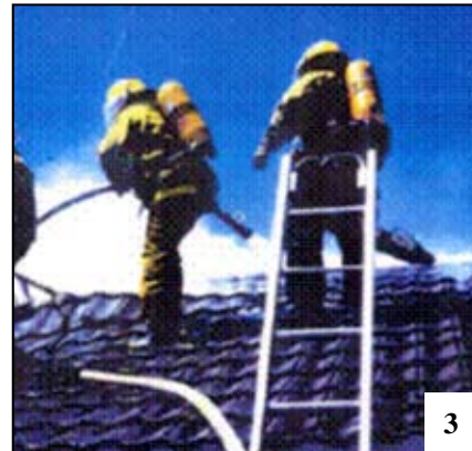
Firefighters on the stone-coated metal roof ventilate the attic by cutting into the roof (but avoid cutting through the rafters) using a carbide-tipped chainsaw with a depth guard set to 3 inches. A slit is cut along the entire ridge line, and then the ridge roofing panels are peeled back to allow water to flow down and inside the roof assembly.
